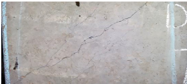
Fig. 2.4. Crack pattern of controlled specimen.
